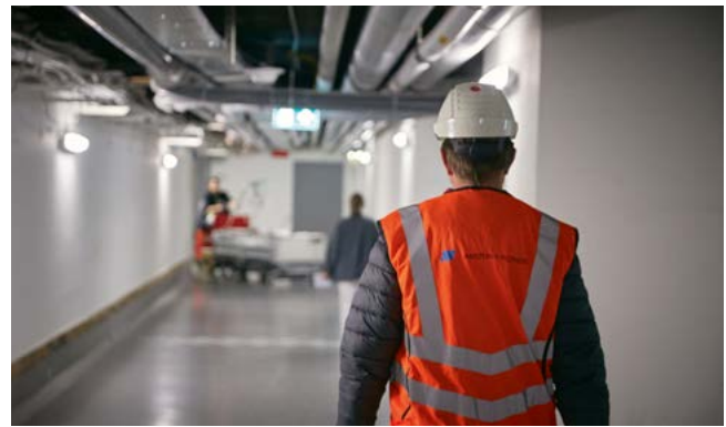
_UNDERGROUND TUNNEL: BUSINESS AS USUAL AT THE HOSPITAL DESPITE THE LARGE CONSTRUCTION SITE.
