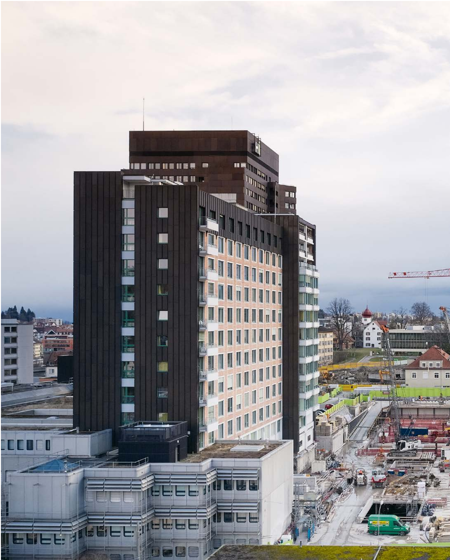
_WORKING IN THE HOSPITAL: THE CANTONAL HOSPITAL IS CURRENTLY ONE LARGE CONSTRUCTION SITE. THE "ONCE-IN-A-GENERATION" PROJECT SHOULD BE COMPLETED IN 2027.
