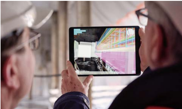
_THANKS TO AUGMENTED REALITY TECHNOLOGY, THREE-DIMENSIONAL MODELS CAN BE VISUALISED DIRECTLY ON THE CONSTRUCTION SITE.
