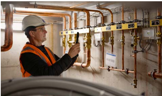
_A QUICK SNAPSHOT, A BRIEF DESCRIPTION AND THE DEFECT AND ITS LOCATION ARE SAFELY LOGGED.
