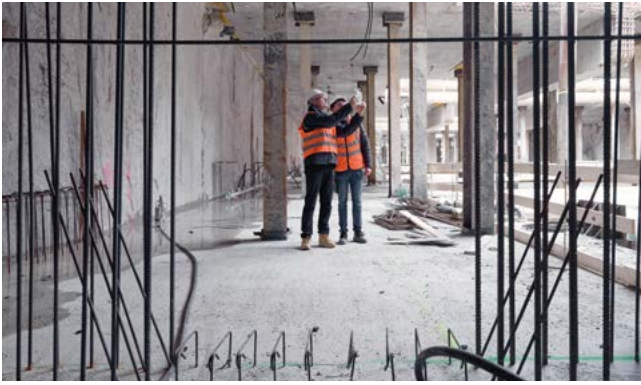
_DIGITAL CONSTRUCTION: THE TOOL CAN HELP BUILDING SITE STAFF COMPLETE VISITS UP TO 50% FASTER.
