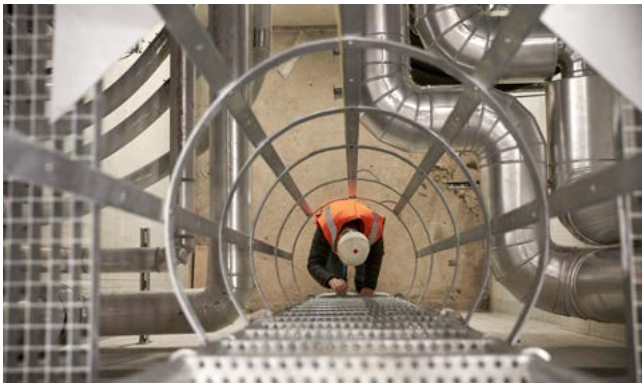
_LARGE CONSTRUCTION SITES ARE HIGHLY COMPLEX AND FULL OF NOOKS AND CRANNIES.
